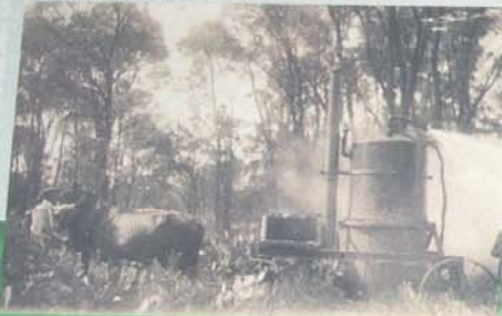
In attempts to destroy prickly pear, it was chopped and covered with sodas and gassed with chlorine and more toxic substances.
